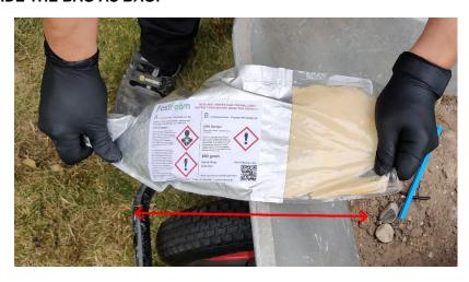
7. To avoid spillage, prior to cutting the bag spout, gently push the product out of the spout first. Tear the bag spout along the tear notch. Always have a knife or scissors ready to cut the spout in case the tear notch fails. Always point the opening in a safe direction as small quantities may leak once the bag has been opened.
