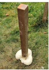
10. Approximately 15-30 minutes after application the excess of PostFoam may be cut off with a saw or with knife. Once the excess has been removed, PostFoam may be topped up with dirt and you can start to build or mount the fence, gate, mailbox or sign.
